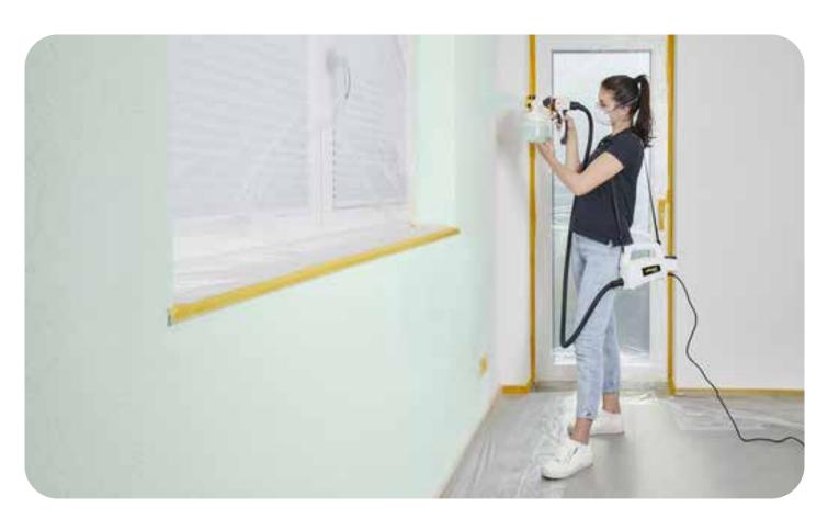
the gun at a 90 degree angle. Paint one square meter at a time. Start at the top and move down.
